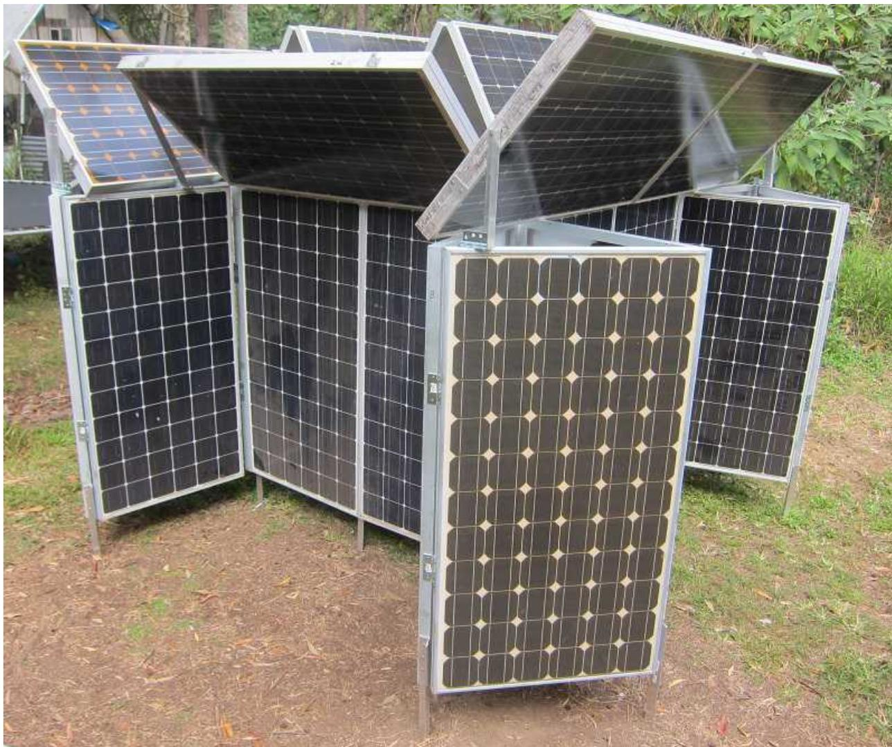
**It is made up of 36 x 195W panels in parallel,** charging 24V 320Ah batteries made up of 8 x 6V 160Ah Maxon Electric Vehicle batteries coupled with a super capacitor.
