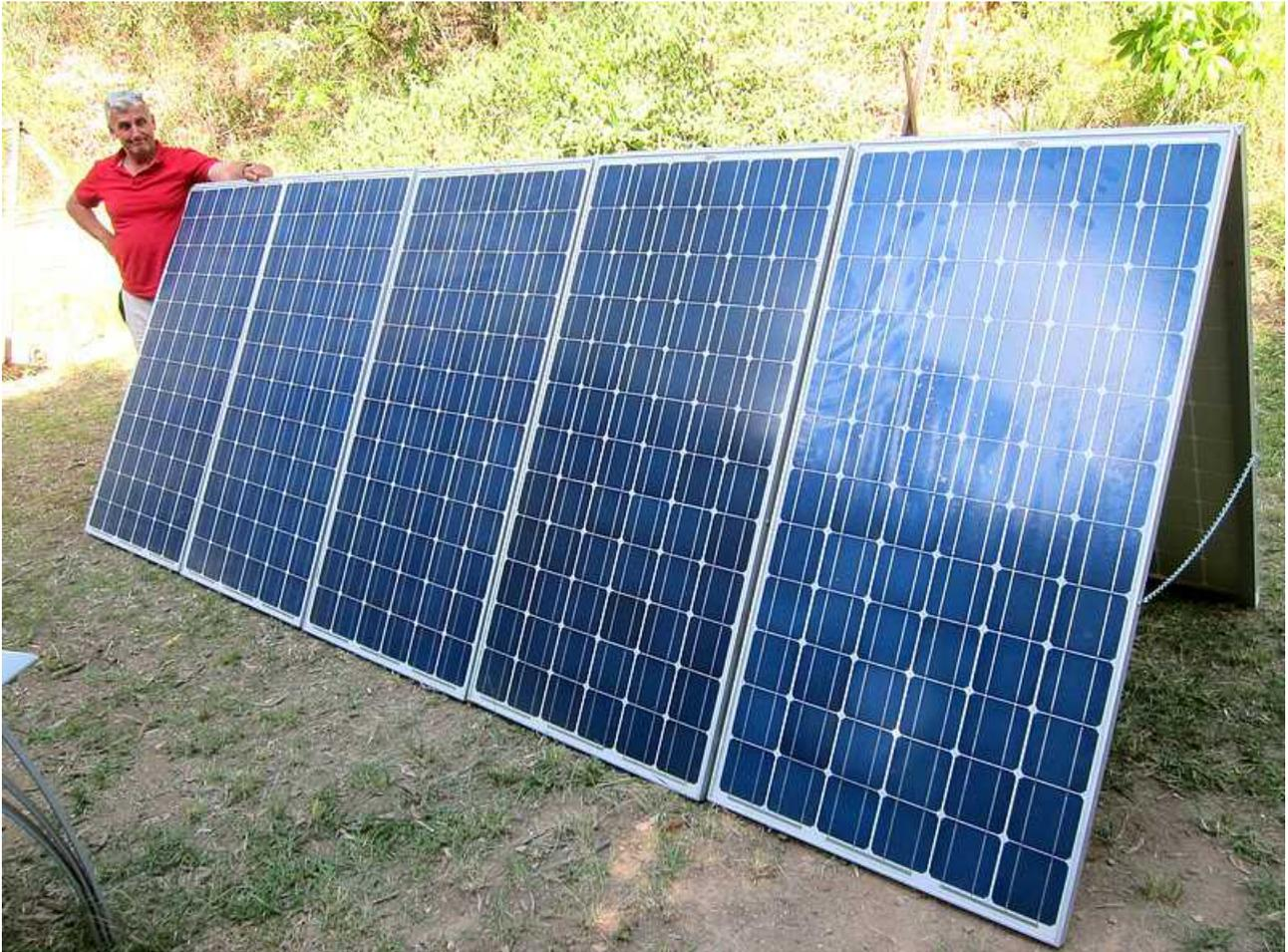
**A-Frames made up of 185-195W panels generally put out around 300W per cloudy day.** This makes calculating the amount of A-Frames required, an easy task.
