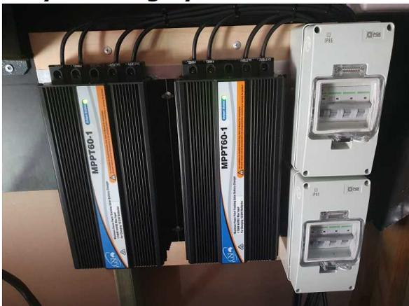
**To make connections easy**, they come mounted and pre-wired with breaker fuses, lugged battery cables and solar panel input plugs.
